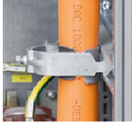
Figure 11-10 Cable clamp example
