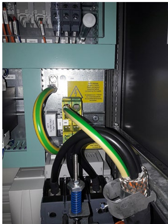
Figure 8-2 Equipment grounding terminals for the incoming supply circuit conductor
