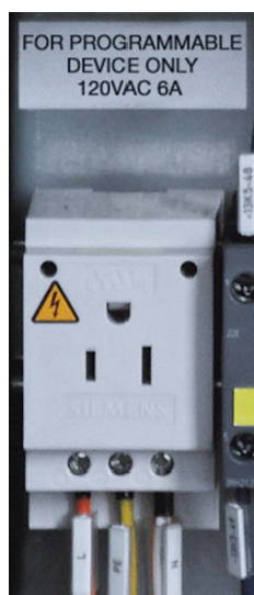
Figure 6-33 Marking of a receptacle
