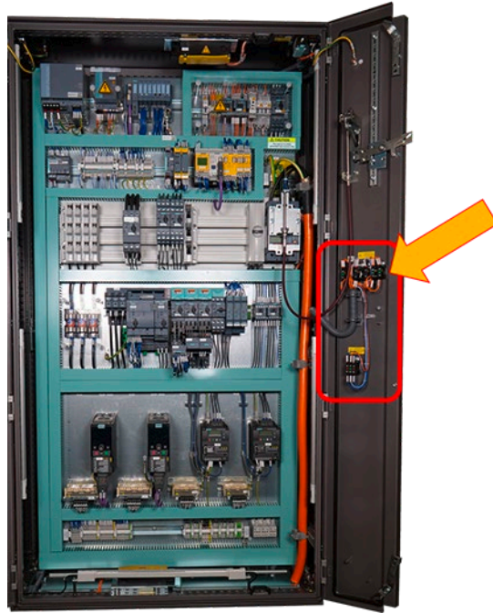
Figure 5-22 Equipment for door mounting
