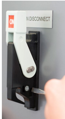
Figure 5-20 Example: Defeating with a screwdriver
